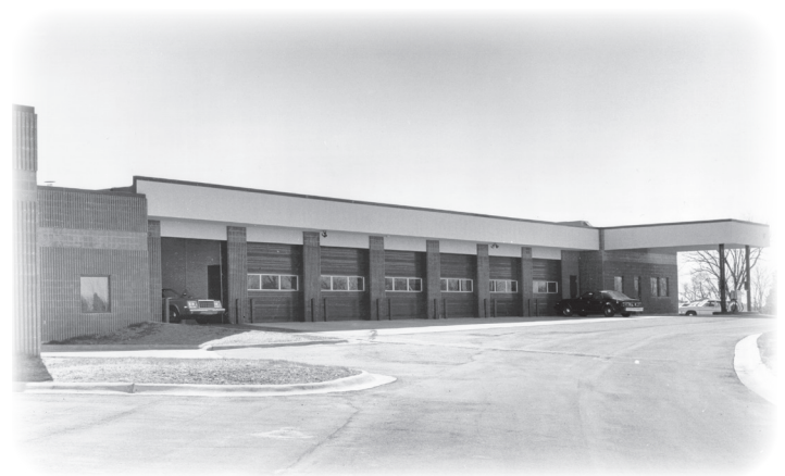
The Patrol Garage and Radio Shop, located behind Troop F Headquarters, were completed in 1981.
