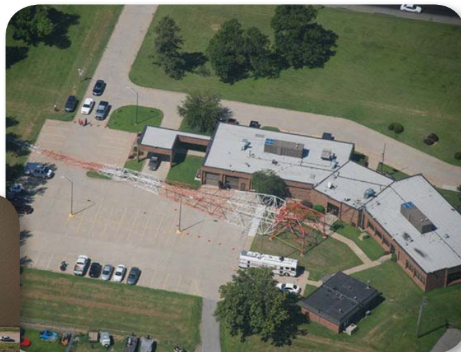
Severe weather took down Troop H's radio tower in 2011.
