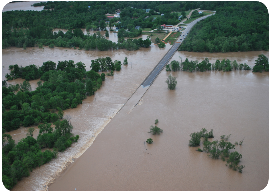
Heavy rainfall caused the Current River to flood over the U.S. Highway 160 bridge in Doniphan, MO.
