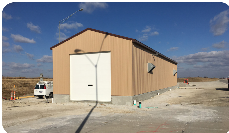
A new inspection building was built at Post H2 South in Harrison County.
