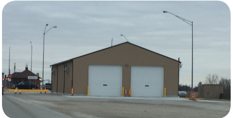
This new inspection building was constructed in Atchison County at Post H4 South.
