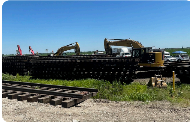
Crews prepare to replace track damaged in the derailment.
