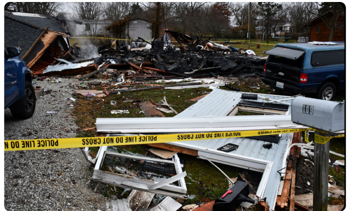
This photo shows the aftermath of a gas leak explosion in Licking, MO.
