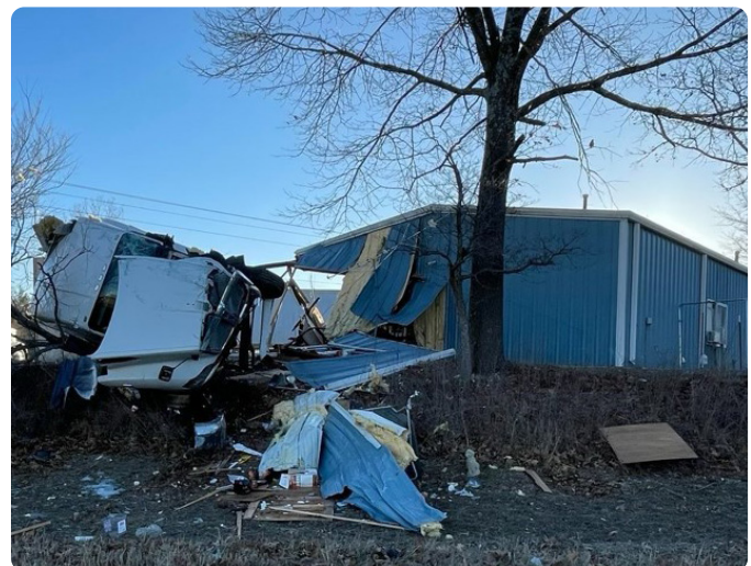
No injuries were reported when this tractor-trailer crashed into a dog-grooming business.
